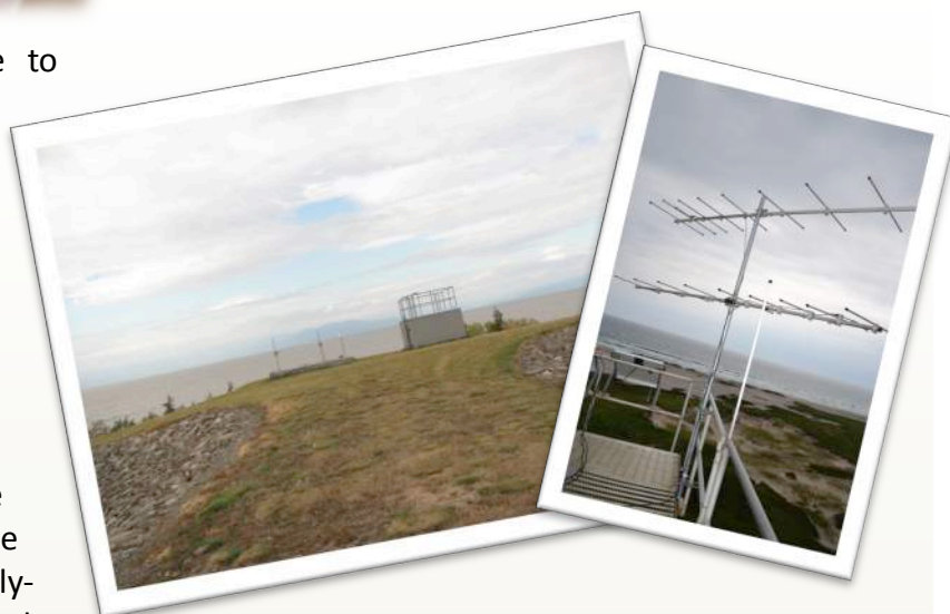
Above Left: Location for new receiving station in St-Jean-Port-Joli, QC. Antennas will be strapped to the cement structure as shown by the picture on the right.
